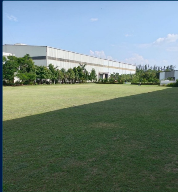
CHINHAT PLANT Lucknow, UP
