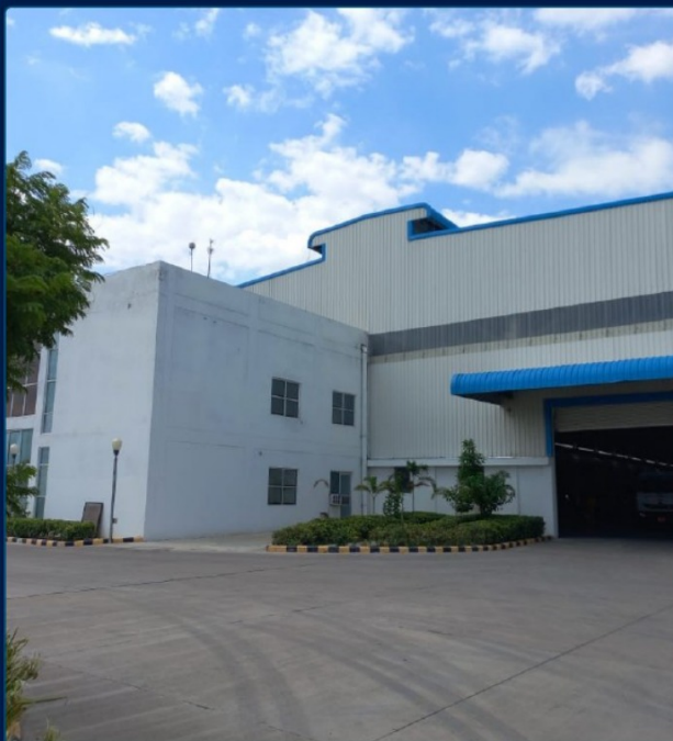
LONG MEMBER PLANT Lucknow, UP
